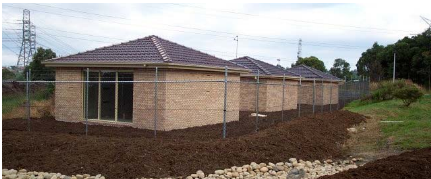
Figure 1-The three building modules for thermal testing
