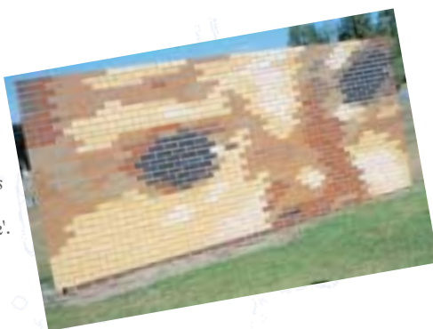
Wordplay: Artist Andrew Leicester drew an analogy with the crossword puzzle. The bricks were stack bonded to achieve the grid with the numbers sand-blasted into the brick face.
