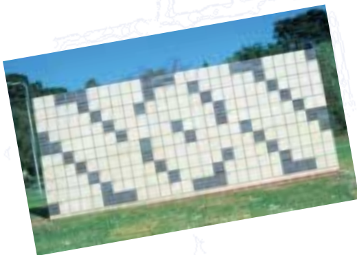
Wordplay: Artist Andrew Leicester drew an analogy with the crossword puzzle. The bricks were stack bonded to achieve the grid with the numbers sand-blasted into the brick face.
