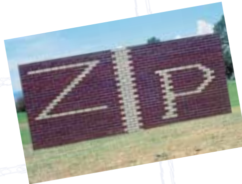
Wordplay: Artist Andrew Leicester drew an analogy with the crossword puzzle. The bricks were stack bonded to achieve the grid with the numbers sand-blasted into the brick face.
