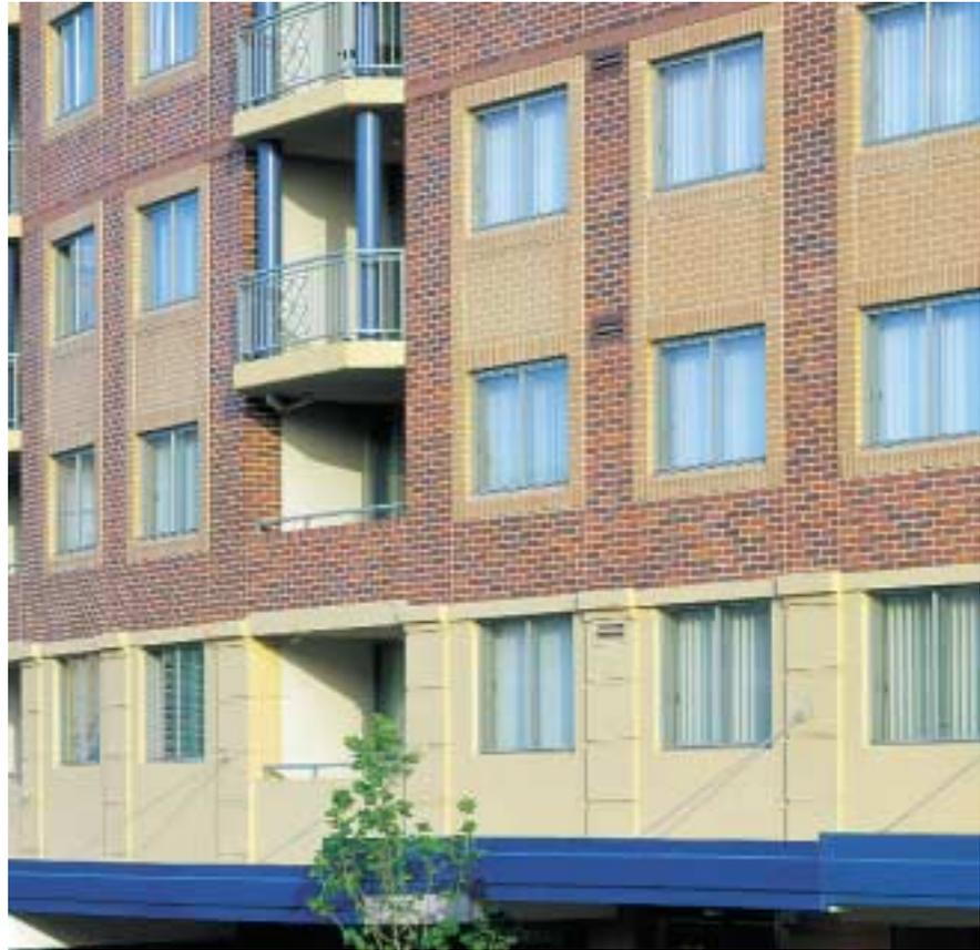
*Face brickwork features above the second level with tan brick panels linking levels. Note the neatly detailed reveals.*
