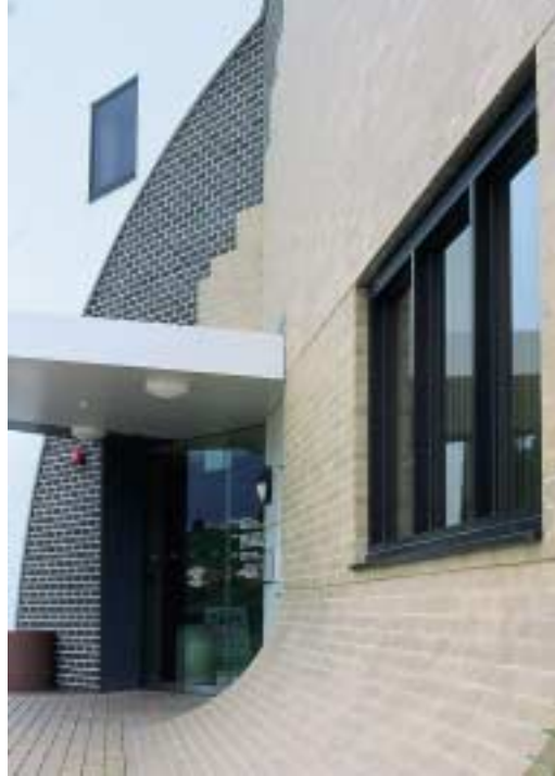
(Left) Paving makes a gentle transition to walling at the main entrance. The cream brickwork is surmounted by an arc of darker bricks. (Below) The controversial 'splat' panel: a 'point of erosion' or is this where that wily coyote met yet another untimely end? (Bottom) Despite their apparent complexity the patterns were cleverly designed to allow rapid laying.
