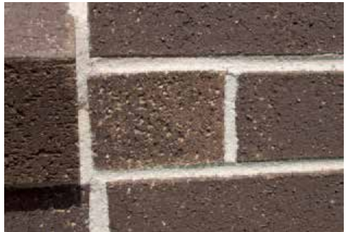
Damage to ironed mortar joint
